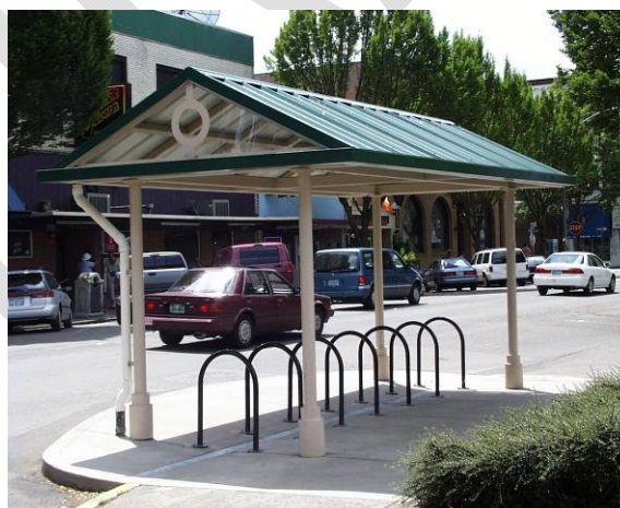
Covered bicycle racks provide protection from rain and other elements.
